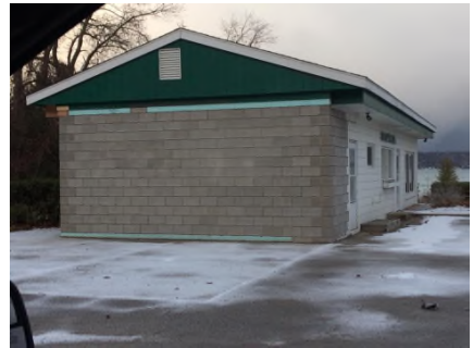
The repaired wall, done with concrete.
